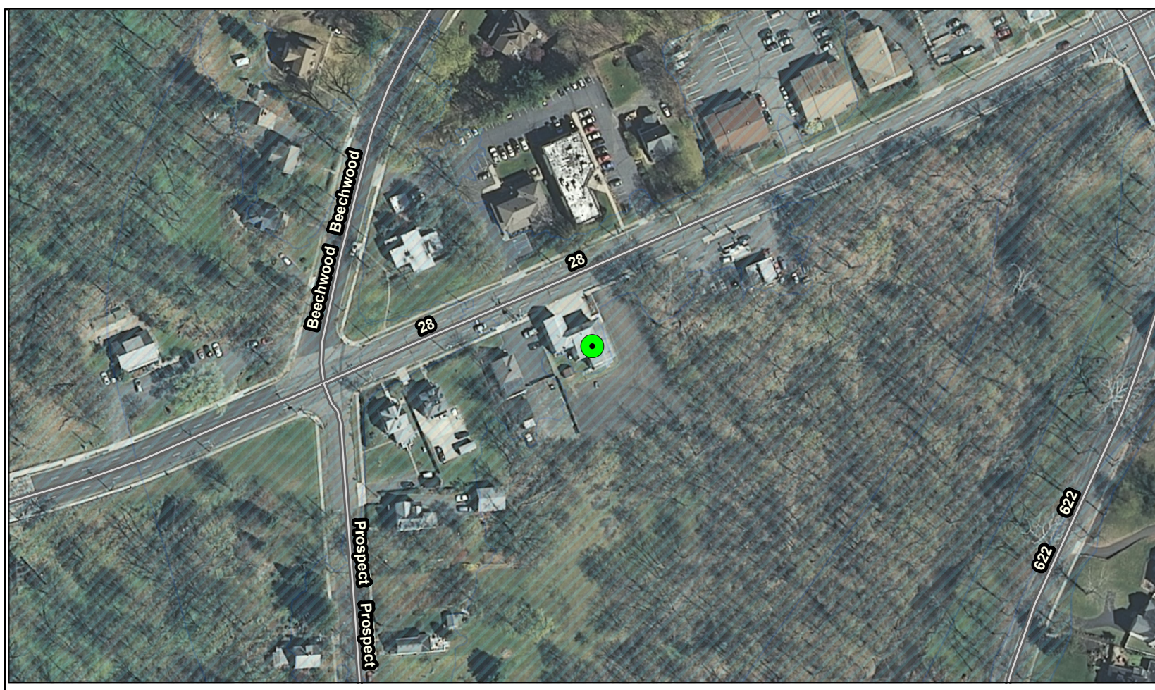
Beechwood Heights Fire Company is an At Risk Essential Facility located in the floodplain.
