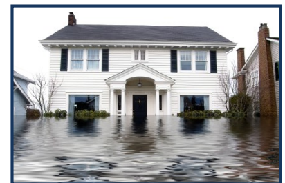
Clusters of past flood insurance claims can show where there is a repetitive flood problem.
