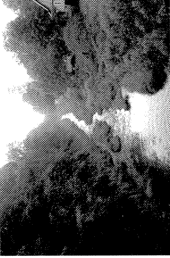
8. Looking D/S from the Davis St. Bridge. Remove sediment bars. Cut the vegetation in the channel.
