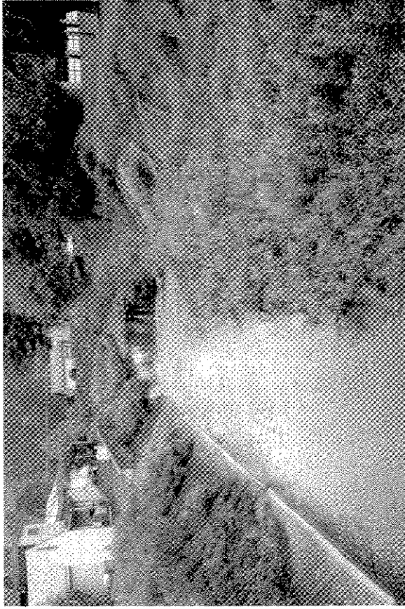
1. Looking D/S from the Main St Bridge. Remove vegetation and sediment bars in the channel.
