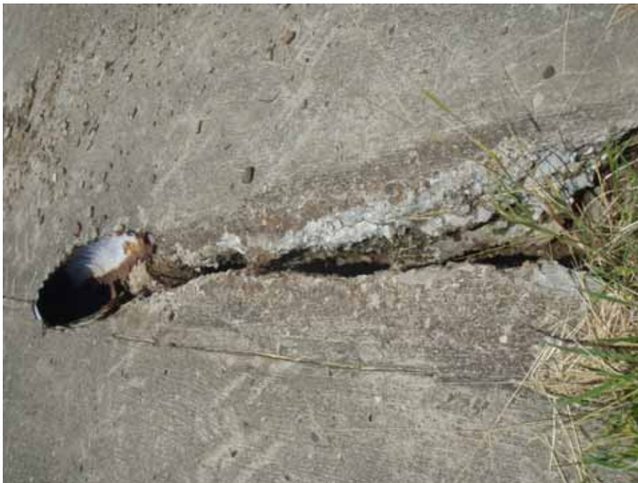
0223: Deep cracks in concrete (U) Near Sta. 47+00
