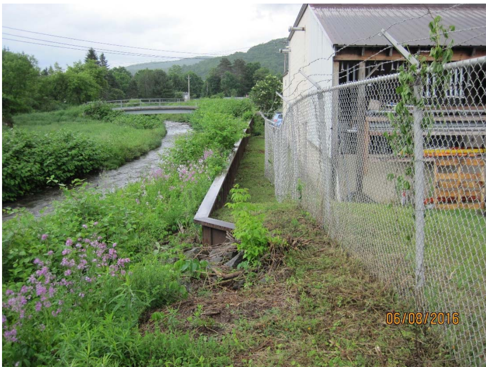
Photo 9: Looking downstream along the sheetpile floodwall portion of the Big Hollow Creek Levee.
