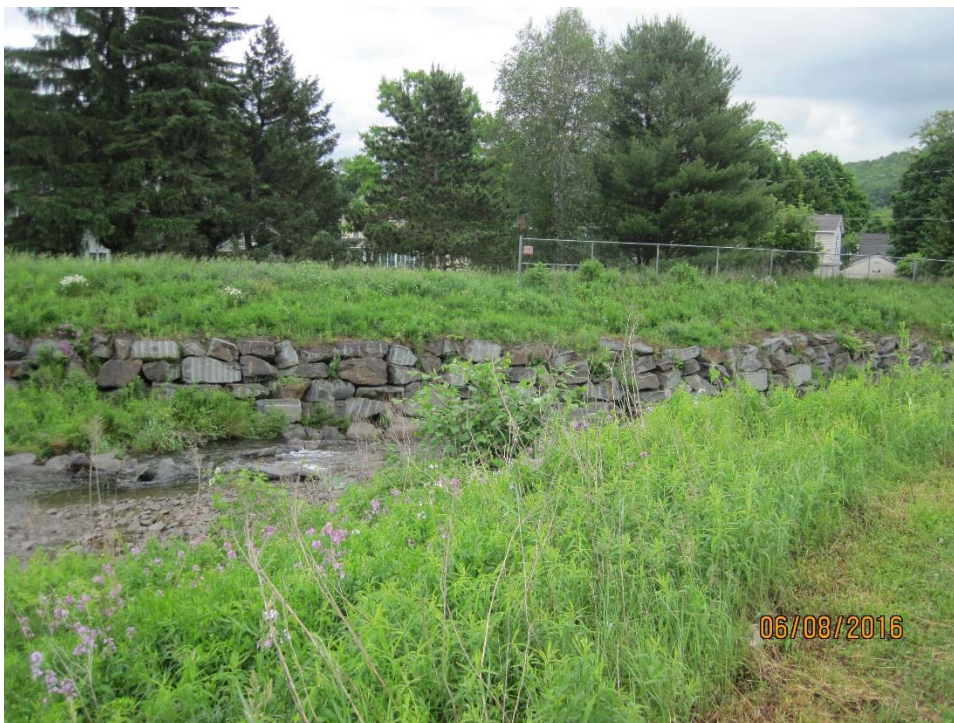
Photo 11: Repaired scarp area on the Butler Brook Levee just upstream from the transition structure.
