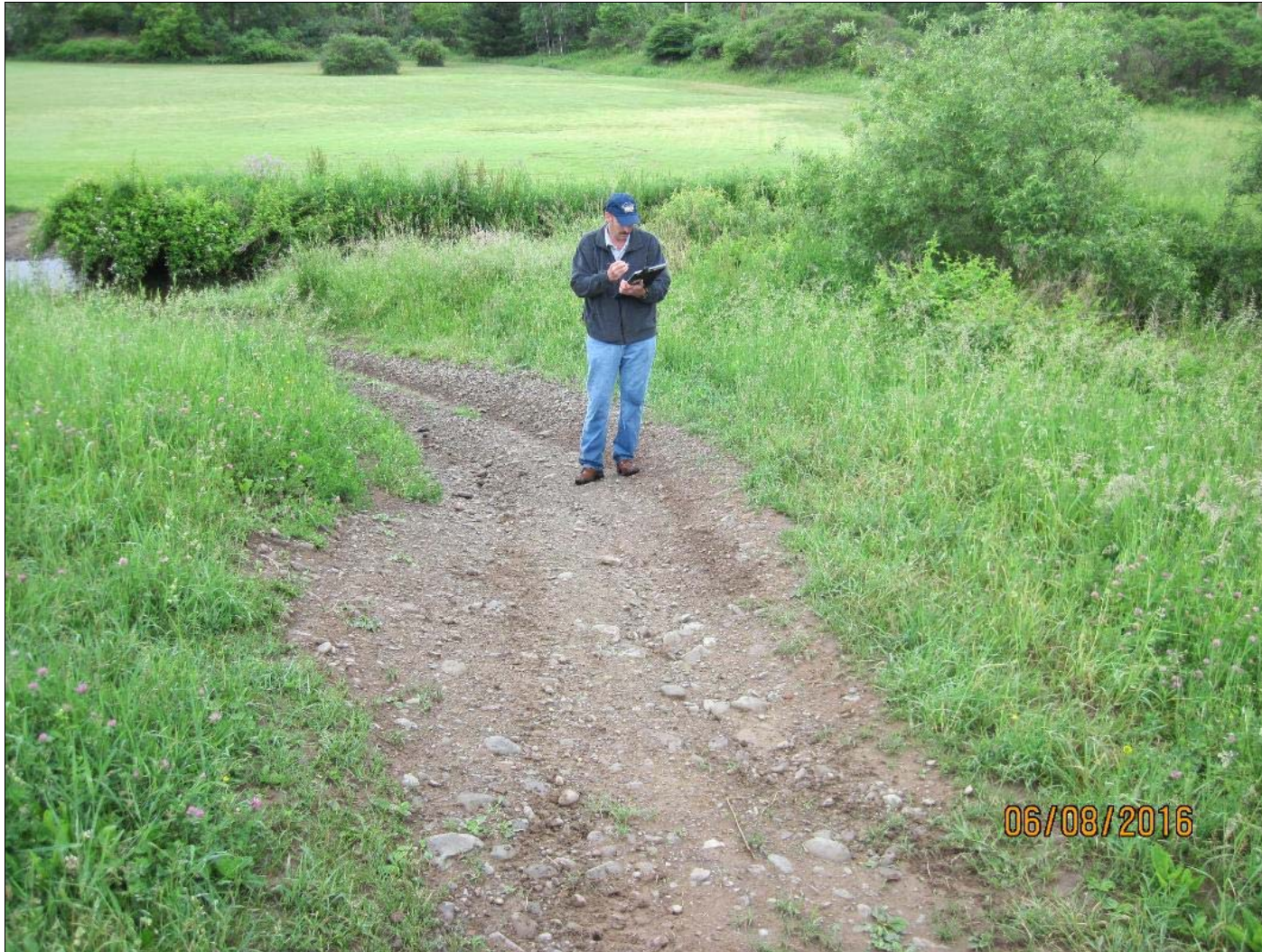
Photo 4. Inspect ID: DEPO_2016_a_0006 Title: USACE_CENAP_DEPO_2016_a_0006_1.jpg Rated Item: 8. Depressions/ Rutting. Caption: Rutting of the riverside slope of the Butler Brook Levee where foot traffic and ATVs pass through.
