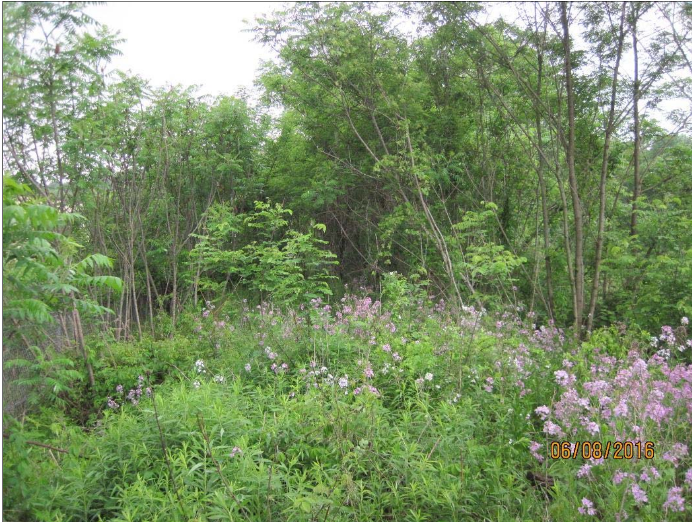
Photo 1. Inspect ID: DEPO_2016_a_0001 Title: USACE_CENAP_DEPO_2016_a_0001_1.jpg Rated Item: 1. Unwanted Vegetation Growth. Caption: Excessive vegetation on the Big Hollow Creek Levee.
