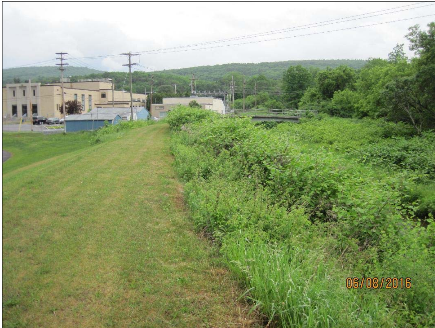
Photo 2. Inspect ID: DEPO_2016_a_0003 Title: USACE_CENAP_DEPO_2016_a_0003_1.jpg Rated Item: 1. Unwanted Vegetation Growth. Caption: Looking upstream along the Big Hollow Creek Levee. Excessive vegetation on the riverside slope.
