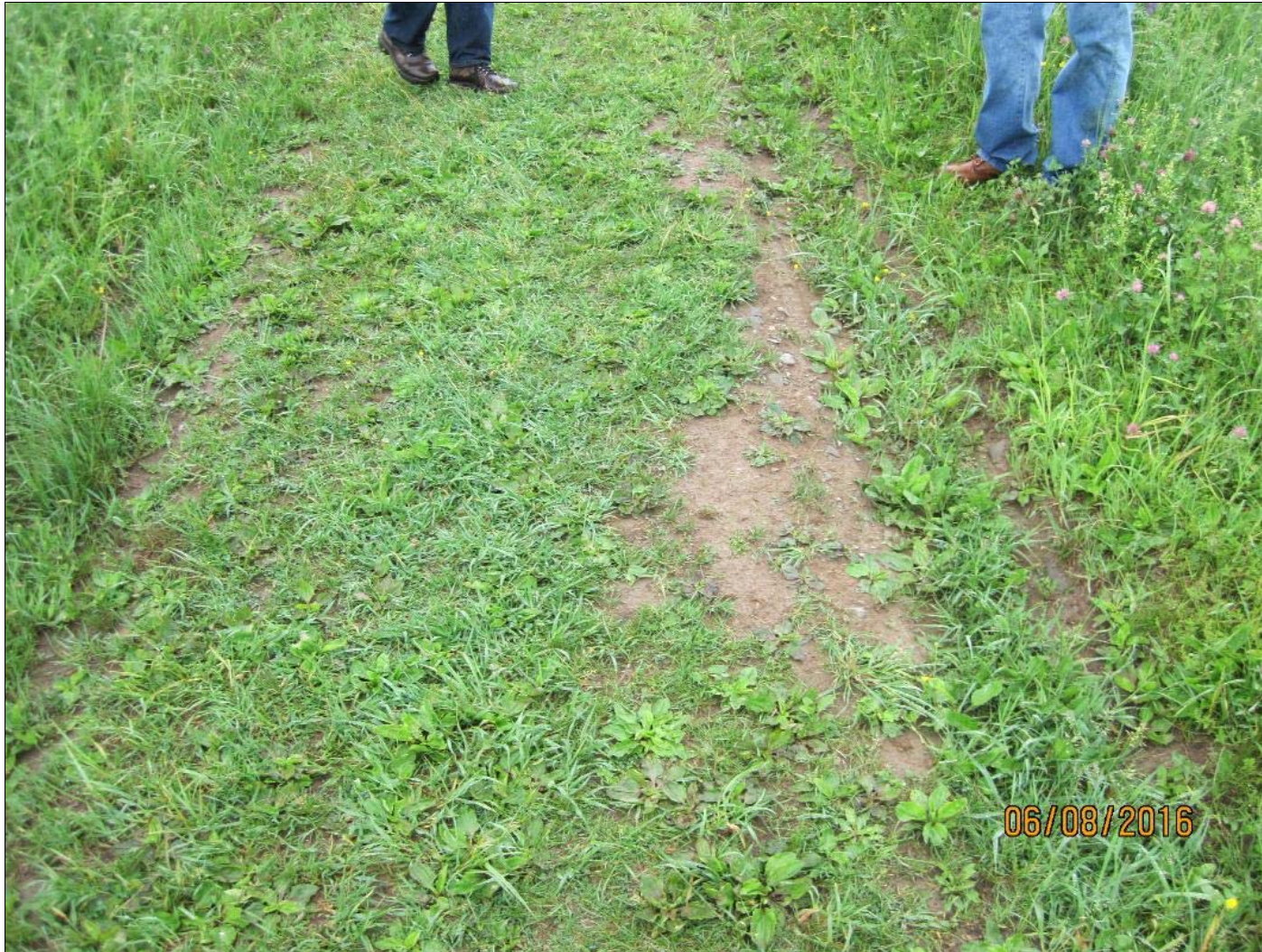
Photo 3. Inspect ID: DEPO_2016_a_0005 Title: USACE_CENAP_DEPO_2016_a_0005_1.jpg Rated Item: 8. Depressions/ Rutting. Caption: Rutting on the Butler Brook Levee crest that was not repaired.
