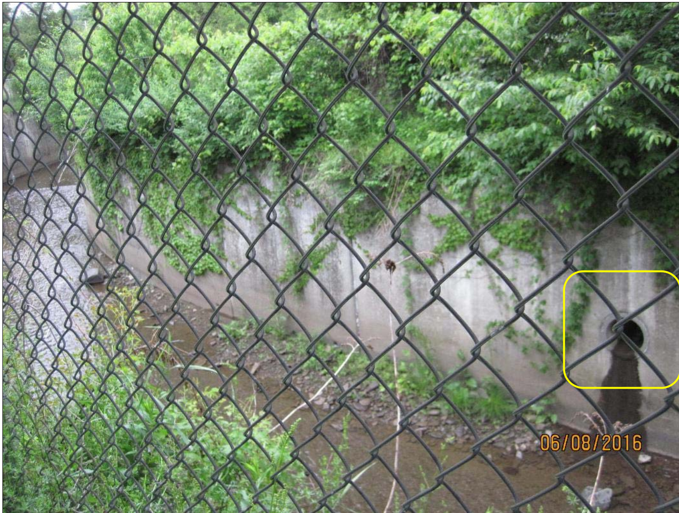
Photo 5. Inspect ID: DEPO_2016_a_0008 Title: USACE_CENAP_DEPO_2016_a_0008_1.jpg Rated Item: 9. Flap Gates/ Flap Valves/ Pinch Valves. Caption: Drainage pipe exiting into the diversion channel.
