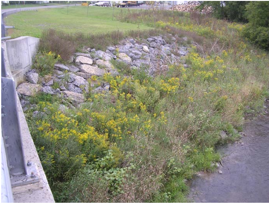
Photo 21: Vegetation in riprap at West Cayuga Street bridge, Owasco Inlet.
