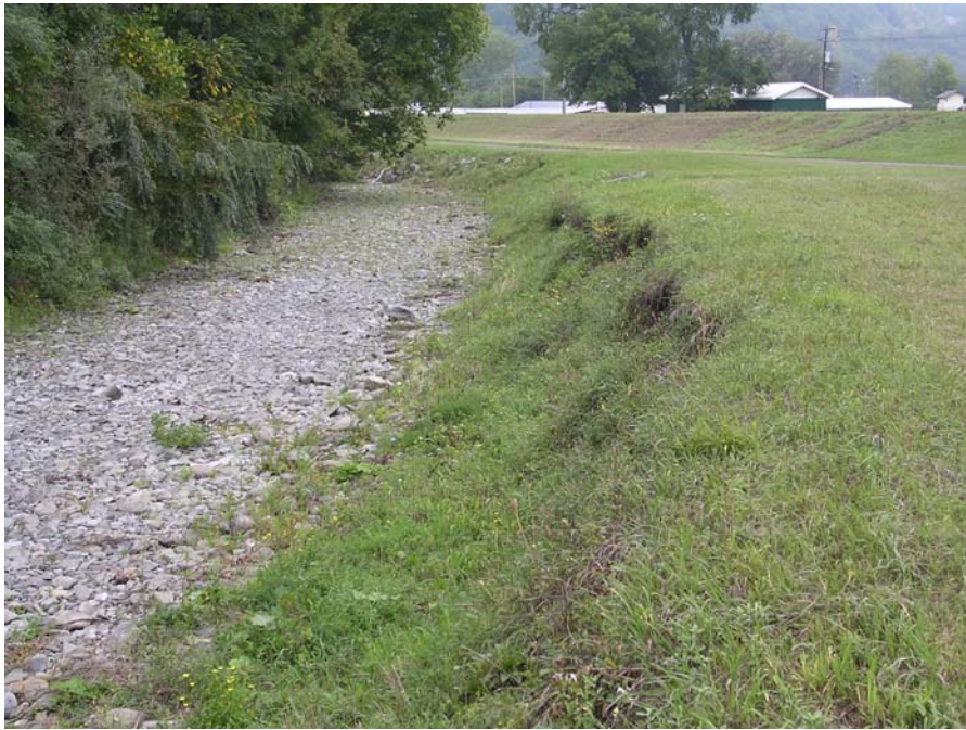
Photo 5: Erosion along right bank of Dry Creek between Route 38 and abandoned Lehigh Valley Railroad bridge.
