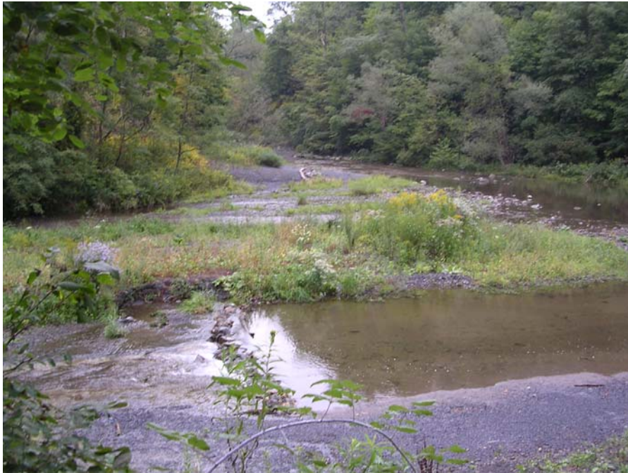
Photo 12: Mill Creek settling basin. A moderately large vegetated shoal has developed in middle of settling basin.
