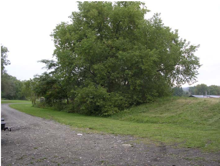
Photo 8: End of levee near abandoned Lehigh Valley Railroad bridge – levee is open ended at this point.
