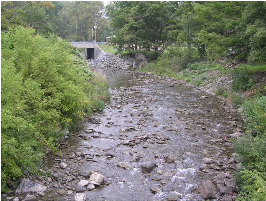
Photo 13: Looking upstream at Mill Creek from Smith Street bridge. Vegetation growing in the riprap along the left and right banks.
