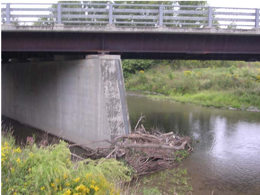
Photo 20: Debris accumulation on the upstream side of the West Cayuga Street bridge, Owasco Inlet Channel.
