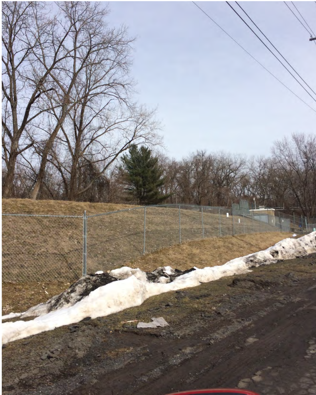
Kingston Levee Looking East to Pump Station
