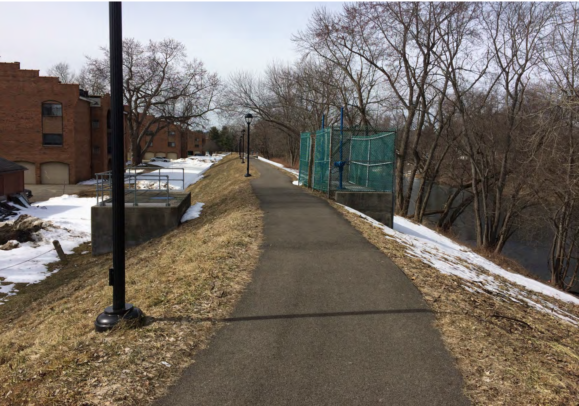
Kingston Levee Looking West Behind Apartments
