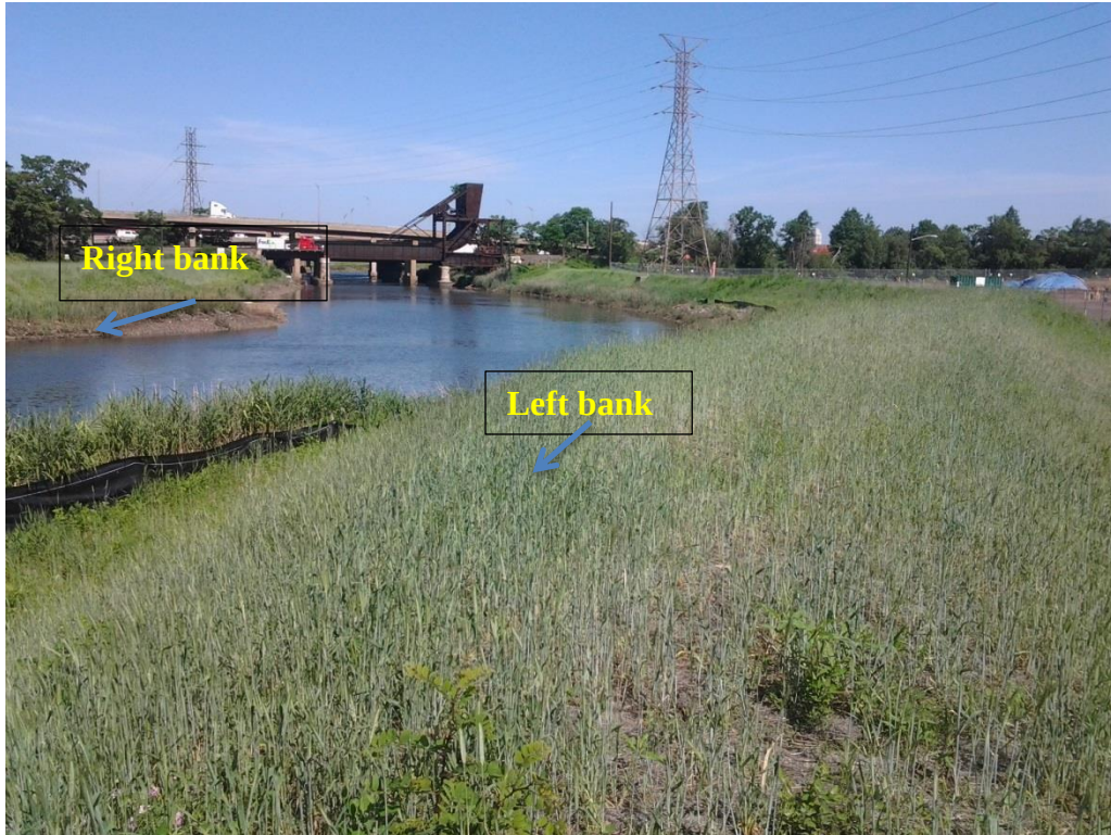
Figure 3: Left and right banks of the Elizabeth Levee looking upstream toward the railroad bridge
